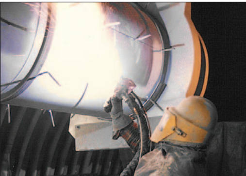
Cathodic protection, thermally sprayed aluminum, reactor silencer, Toronto
