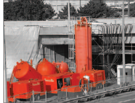
Lead paint remediation and abatement and plural component coating application, Dixon Rd. and Hwy. 401, Toronto, Ministry of Transportation Ontario
