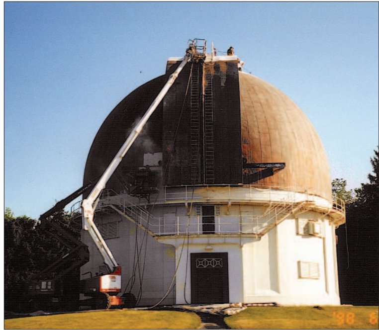
Water blasting and protective high performance coating application on copper metal, David Dunlap Observatory, Toronto
