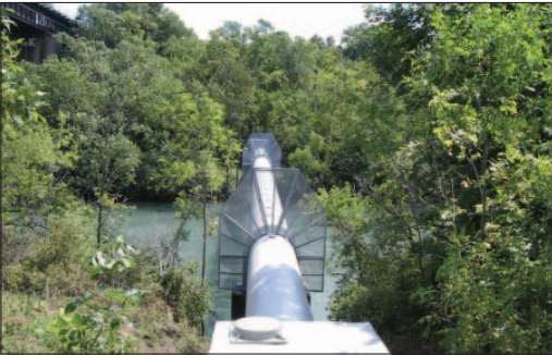
Protective coating application and upgrading of elevated sewer crossings, Niagara Power Canal, St. Catharines Municipal Golf Course
